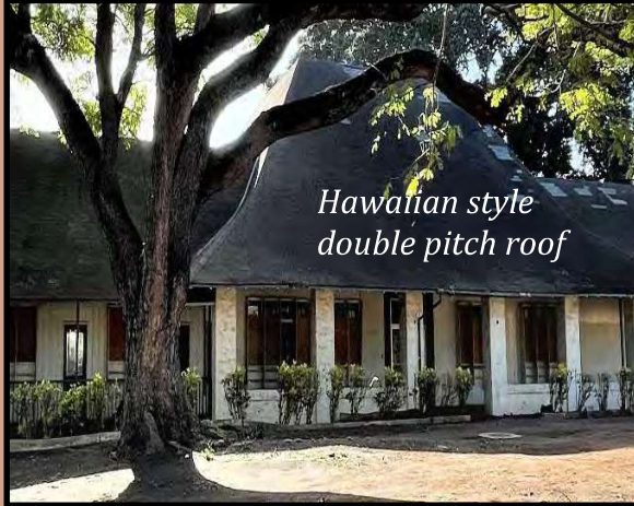
Figures 23 & 24: Main façade – west elevation of the Waiialua Sugar Company Administration Building exhibits the Hawaiian style double pitch roof (Left); North view of the stucco finish columns, connecting stucco wall with weep holes and bench seating. (Right).
