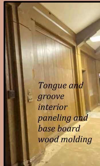
Figures 48 & 49: Interior of the accounting office featuring carved decorative wall trim with a diamond fret pattern (Left); and tongue and groove interior siding and base board wood molding (Right). Source: FAI Architects, 2023
