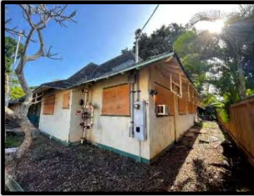
Figure 77: Boarded up windows with plywood.
