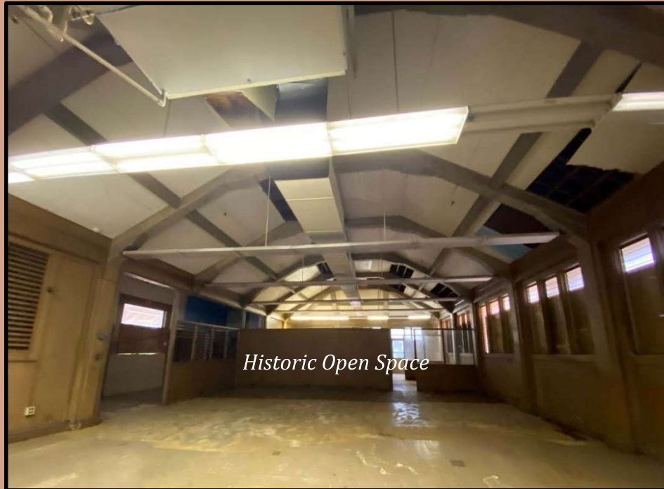
Figure 45: Interior of the accounting office historic open space featuring exposed truss ceiling. Non-original fluorescent lighting. Source: FAI Architects, 2023
