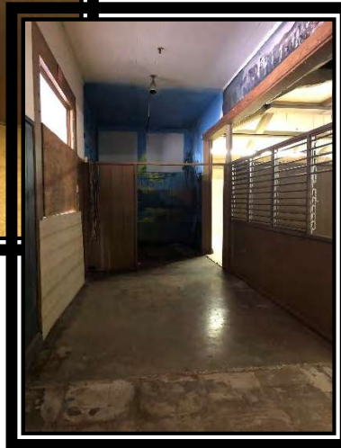
Figure 99: Entrance lobby Source: FAI Architects, 2023
