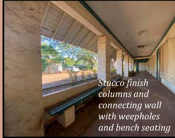
Figures 23 & 24: Main façade – west elevation of the Waiialua Sugar Company Administration Building exhibits the Hawaiian style double pitch roof (Left); North view of the stucco finish columns, connecting stucco wall with weep holes and bench seating. (Right).
