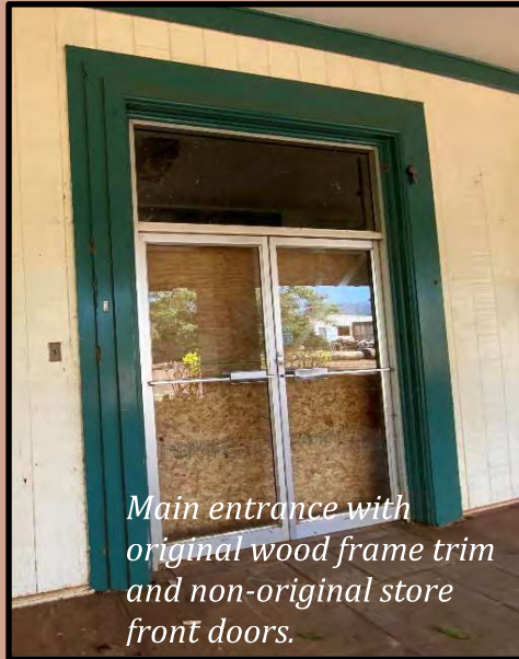
Figures 27 & 28: Located on the main façade – west elevation of the Waialua Sugar Company Administration Building main entrance with original wood frame trim (Left); Single door with glass panel, wood paneling and original hardware (Right).
