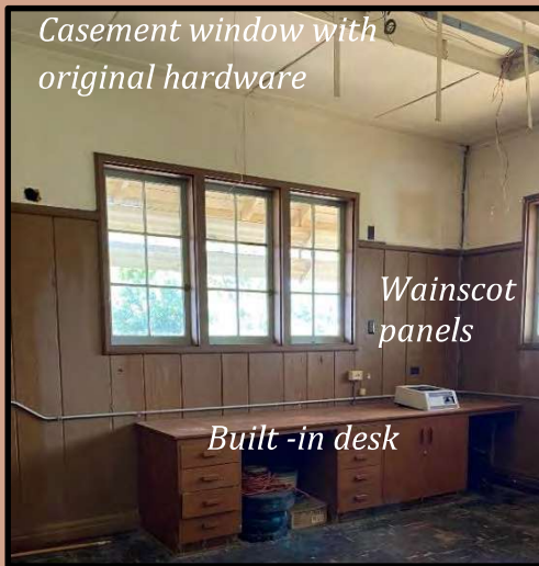
Figures 39 & 40: Interior of the conference room displays built-in desk, wainscot panels and casement windows with original hardware (Left); and built-in storage and sliding door with decorative trim (Right).
