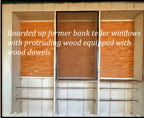
Figures 31 & 32: Located on the main façade – west elevation of the Waialua Sugar Company Administration Building is boarded up former bank teller windows with wood dowels below used to hang work boots during the sugar mill days (Left); Boot scraper (Right).
