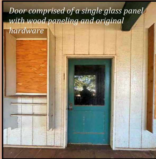
Figures 27 & 28: Located on the main façade – west elevation of the Waialua Sugar Company Administration Building main entrance with original wood frame trim (Left); Single door with glass panel, wood paneling and original hardware (Right).
