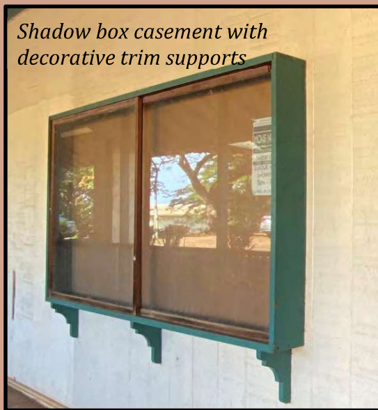
Figures 29 & 30: Located on the main façade – west elevation of the Waialua Sugar Company Administration Building shadow box with decorative trim supports (Left); South view of decorative wood security gate (Right).
